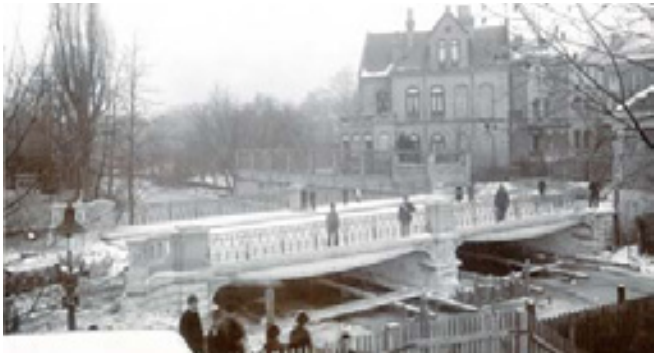
14 Ferdinand-Brücke, Braunschweig, 1901 [TB BS 1.03.11]
