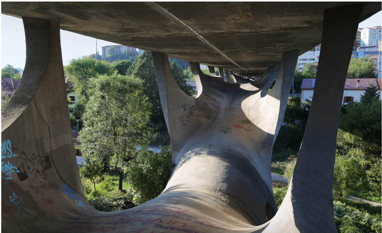
Figure 1: The model-generated form of the Basento Bridge demonstrates the potential of concrete (L. Ingold, 2013).
