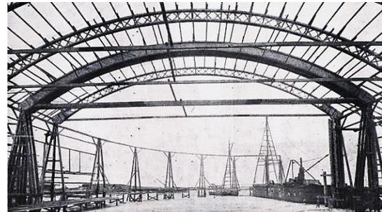
Figure 6: Two-hinge arch with tie (Tuschcherer 1918)
