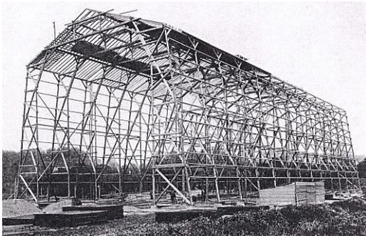
Figure 3: Airship hangar under construction
