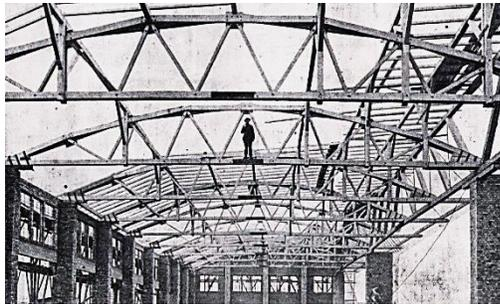
Figure 5: Parabolic truss (Tuschcherer 1918)
